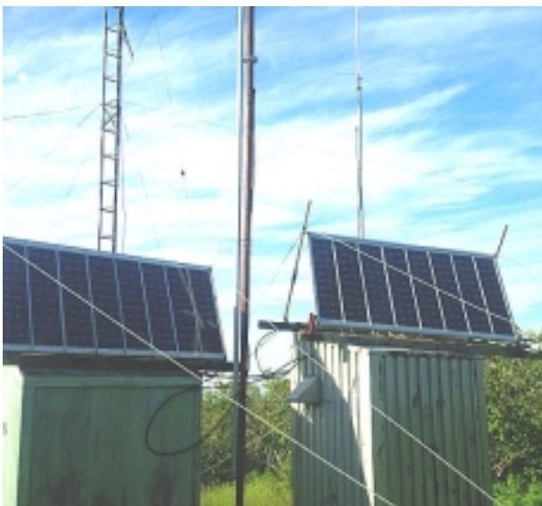
VE1PAR, the Parrsborough 'green' repeater. All solar, it has been running since the nineties.
