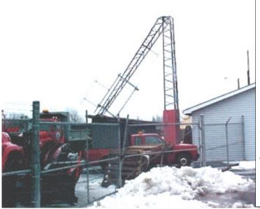
A casualty of the storm which inflicted high winds & snow on Nova Scotia before Christmas was the tower that had been supporting the ham radio antennas at the Yarmouth EOC. Plans are in the works to replace the tower and the bent antennas
